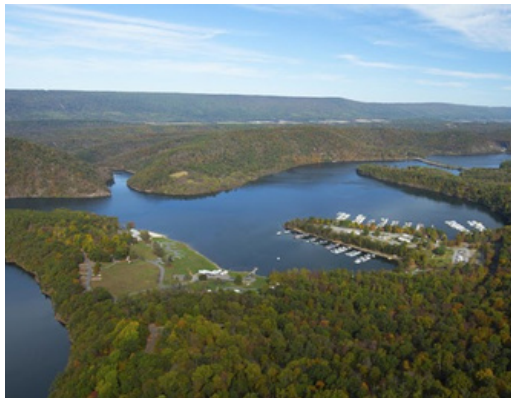
Public Water Supply Reservoir Level Monitoring Network
